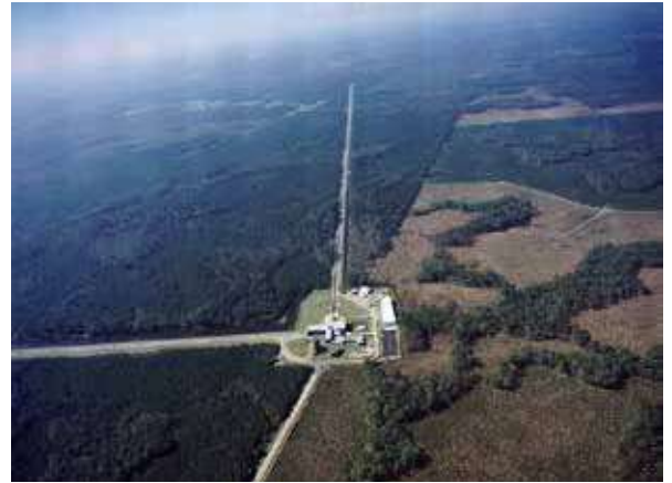
Die LIGO-Anlage in Livingston in Louisiana
